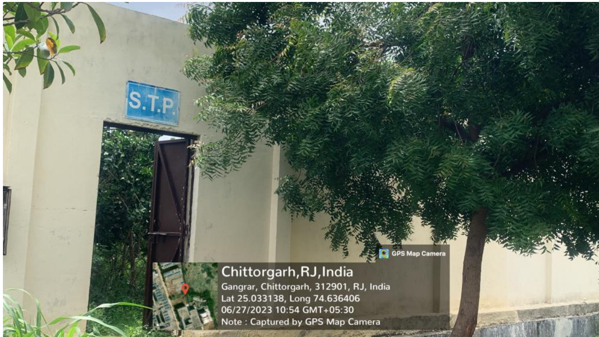
Sewage Treatment Plant
